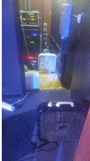
Under roof repair
