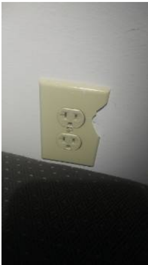
Not tamper proof and broken cover
