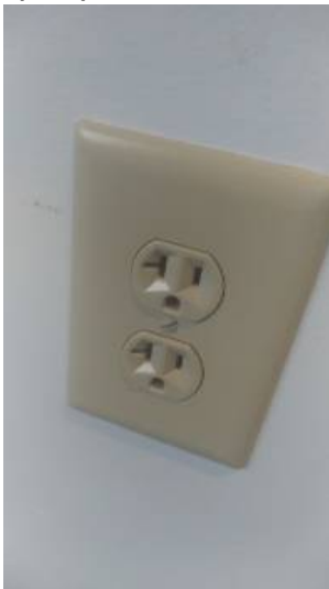
Not tamper proof and broken cover
