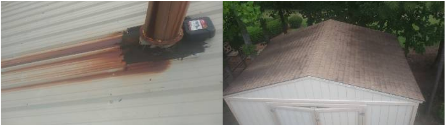
There's a three tab shingle roof on a shed just behind the main building
